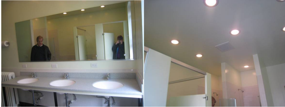
3rd floor bathroom after remodeling
